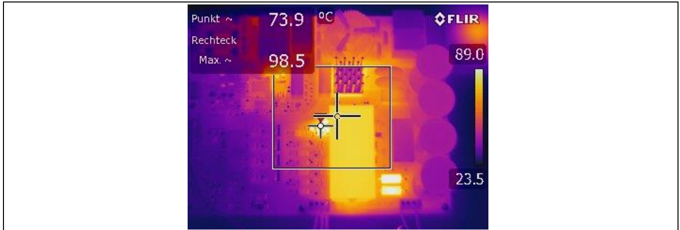
Figure 33 Top view thermal image (hotspot at voltage measurement resistors)
